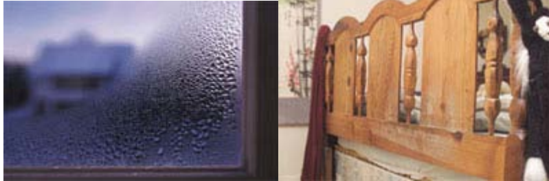
Condensation on the inside of a windowpane. Mold growing on a wooden headboard in a room with high humidity.
